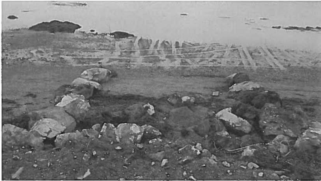
Photos above show the rocks placed around the sewer pipe.
